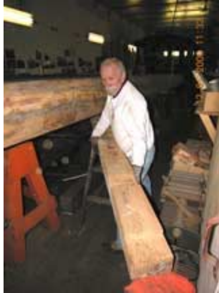
Fred Poore installing needle beam
