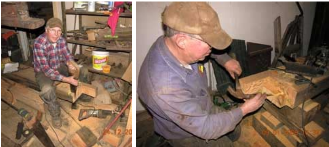
Forming ends of the long sills
