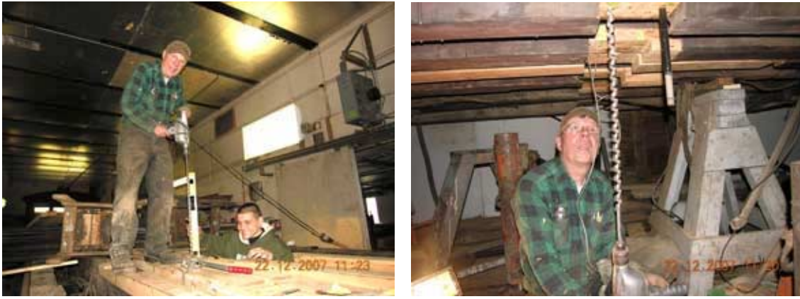
Drilling for bolster bolts with help from Brendan Barlow
