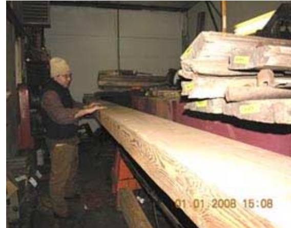
Randy Leclair with ready to upright new sill no. 1
