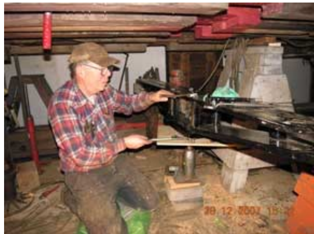
No. 2 end original bolster and Donald Curry installing new one
