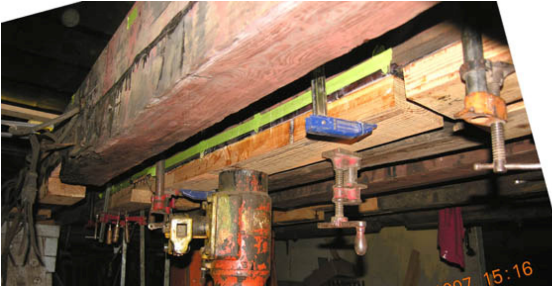
New sill bottom showing jack and many clamps
