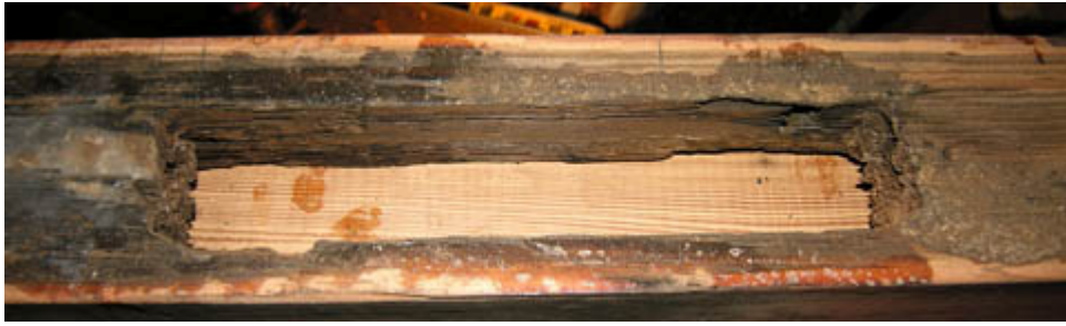
Sill 2 bolt hole area removed-new bottom installed
