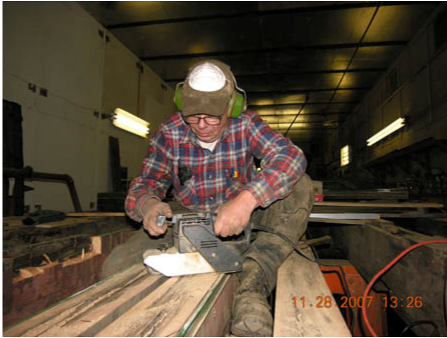
The ex I. S. M. belt sanding the cut-down sill tops
