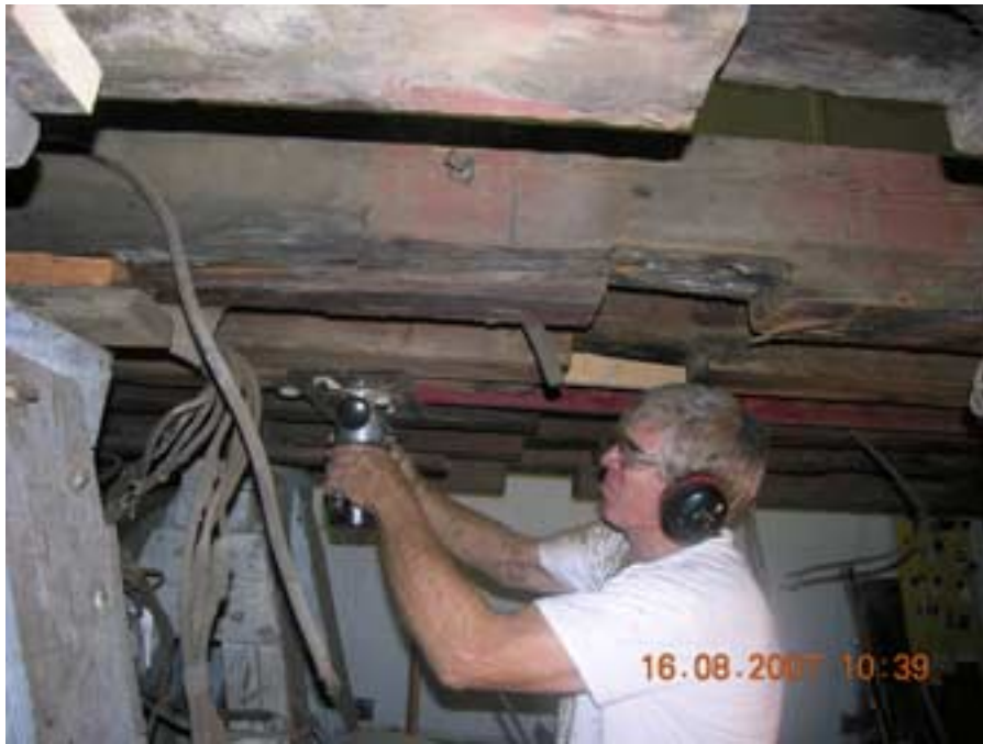
Tom Dow routing out deteriorated wood on bottom of longitudinal sill
