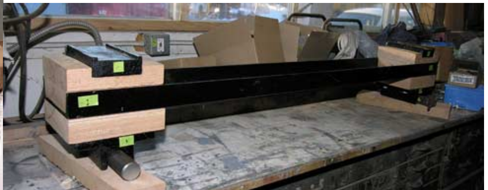
Original and new spring plank assembly (The wood on either side of the top casting had broken away on removal.)
