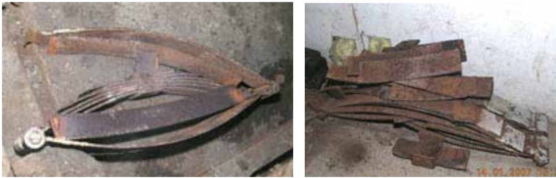
Disintegrated elliptical bolster springs
